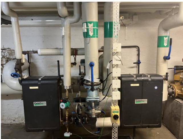
Picture 4: Exemplary substation of residential building in Malmö
